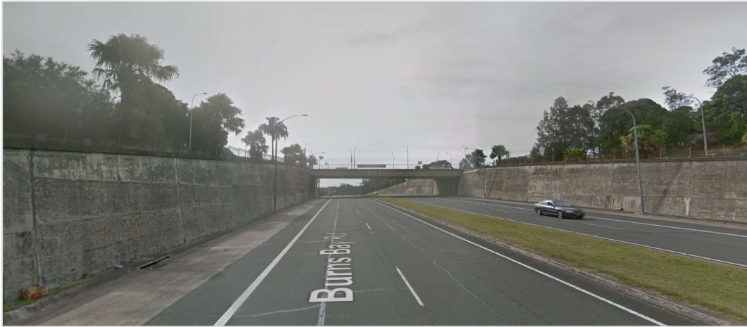
Figure 3: Church Street overpass from Burns Bay Road – view northbound (Source: Google Maps)
